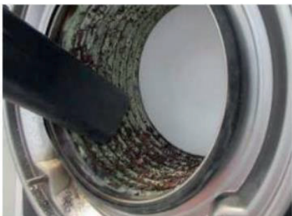
5. Final vacuuming of deposits.
