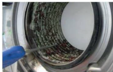
4. Blow out the spaces between the heat exchanger spirals under high pressure.
