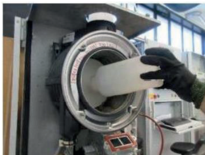
6. Flush the coils of the heat exchanger with water. 7. Check the condensate drainage. 8. Clean the siphon.
